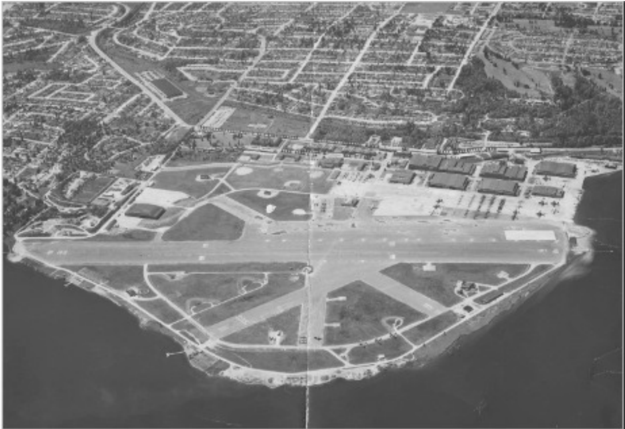
Full build out of Sand Point Naval Air Station with planes on tarmac
